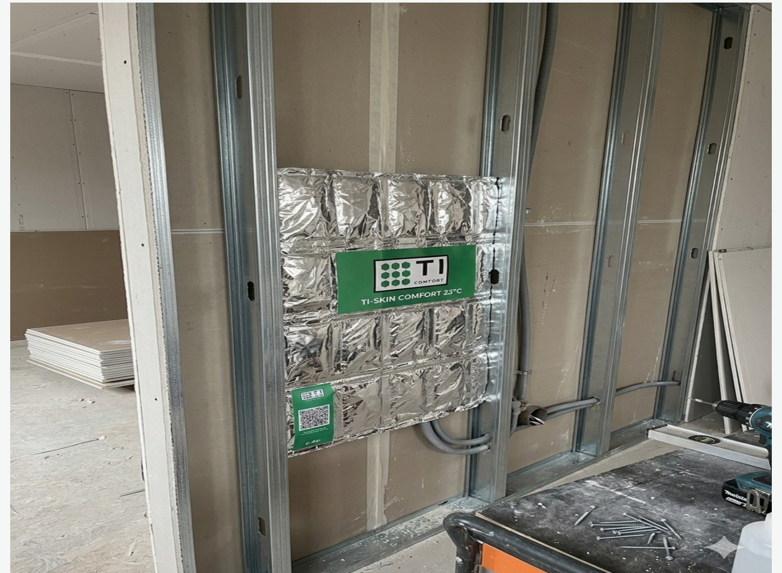
TI-SKIN® installation on site
